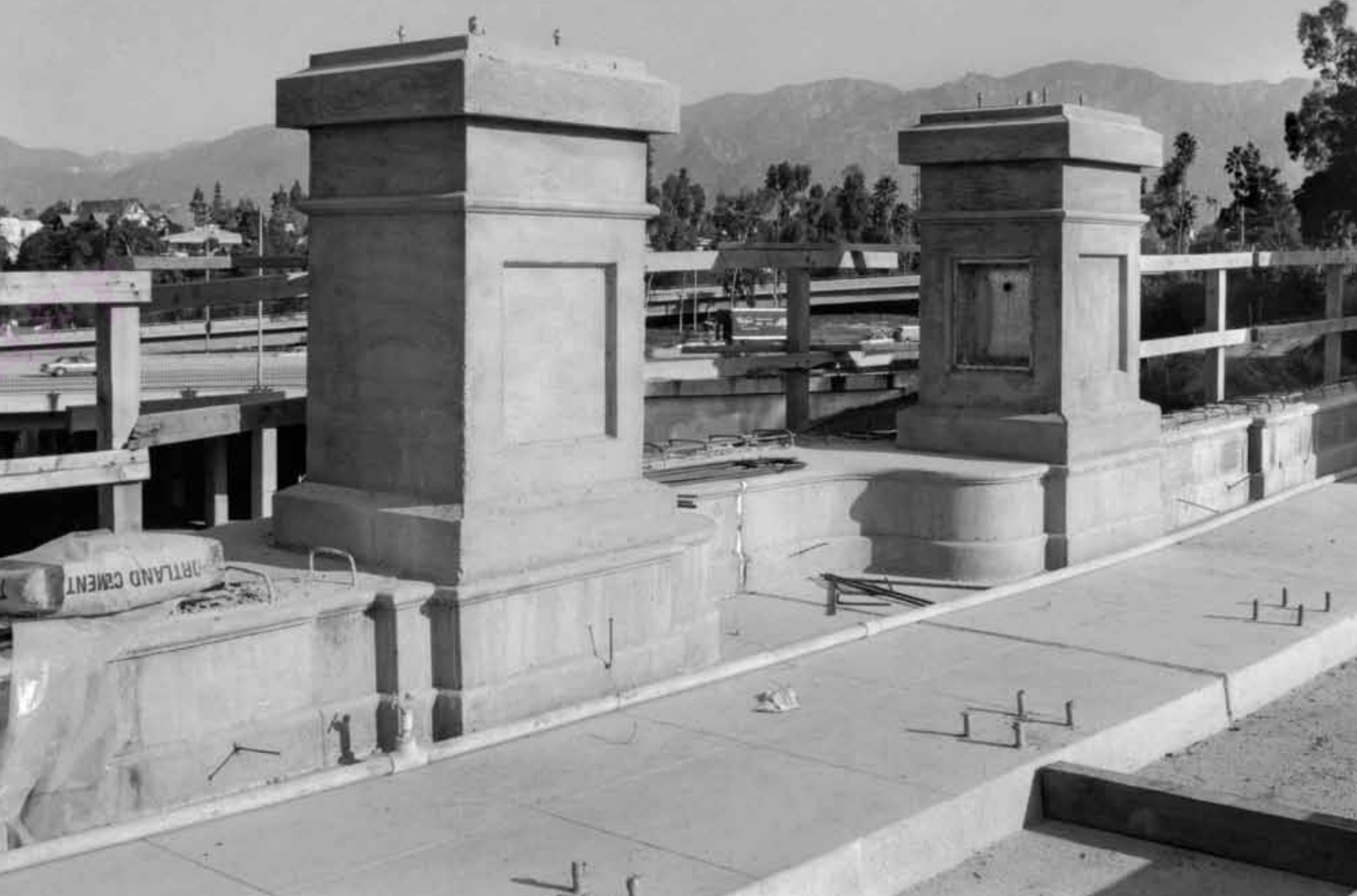
SIDEWALK, BARRIER RAIL, AND LIGHT BASE COLUMNS AFTER STRIPPING FORMS.
