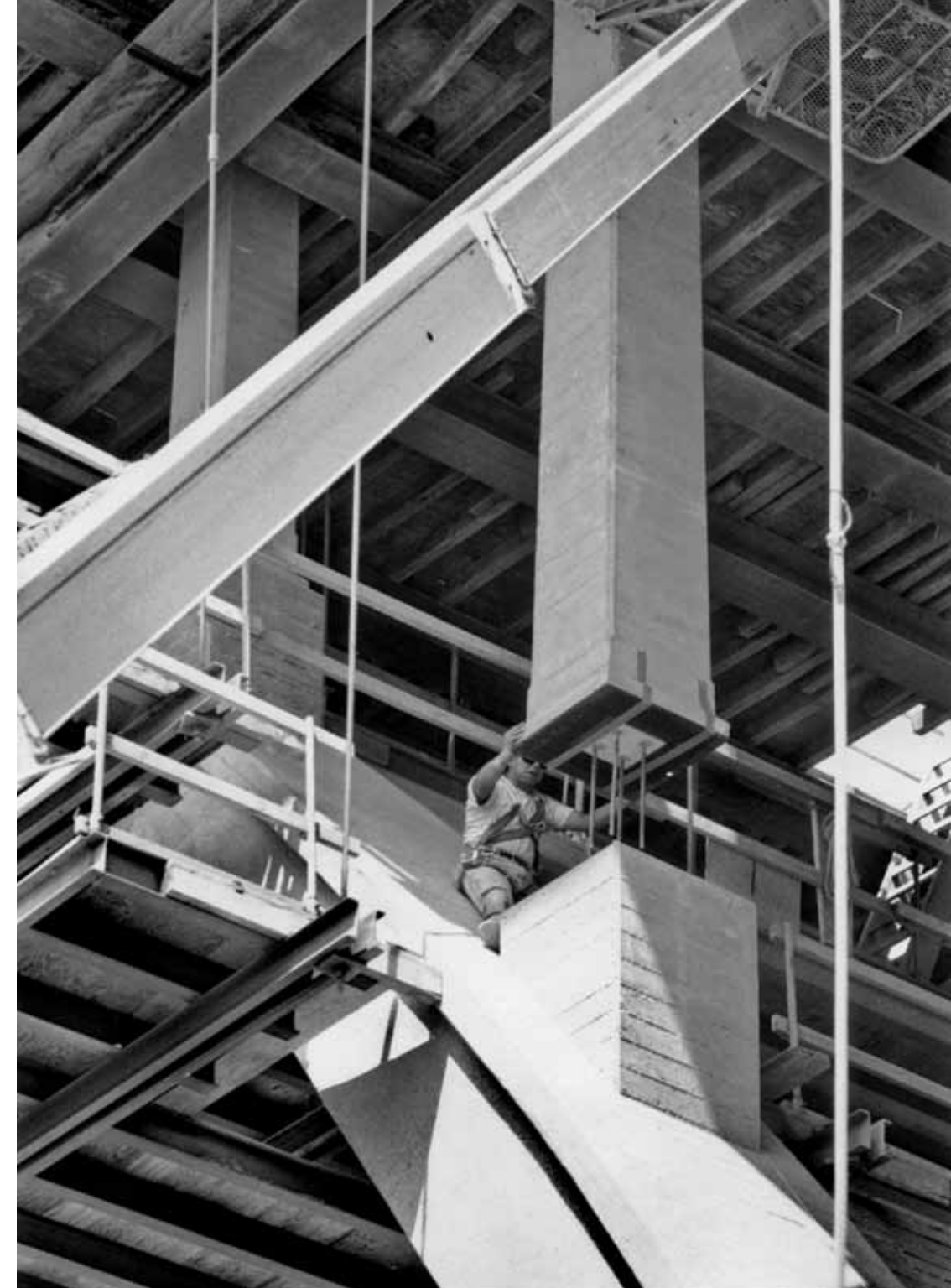
SETTING COLUMN ON NEW CONCRETE BASE.
