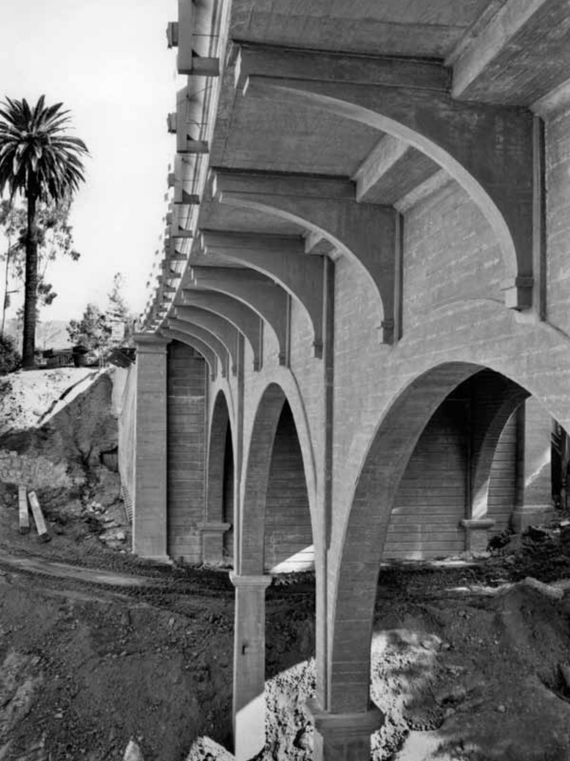
COMPLETED DECK AND OVERHANG SUPPORTS
