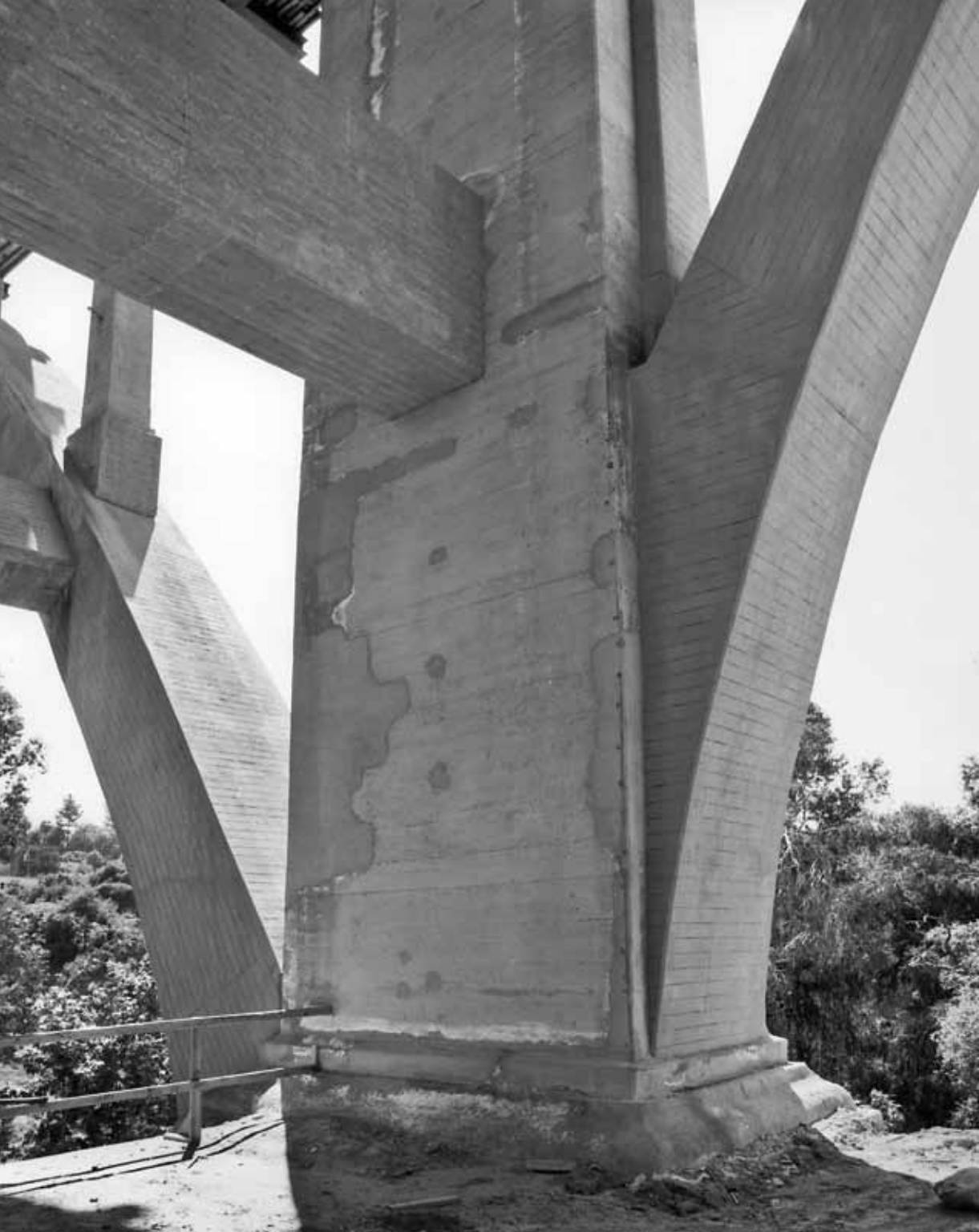
RESTORED BRIDGE PIER @ BASE.
