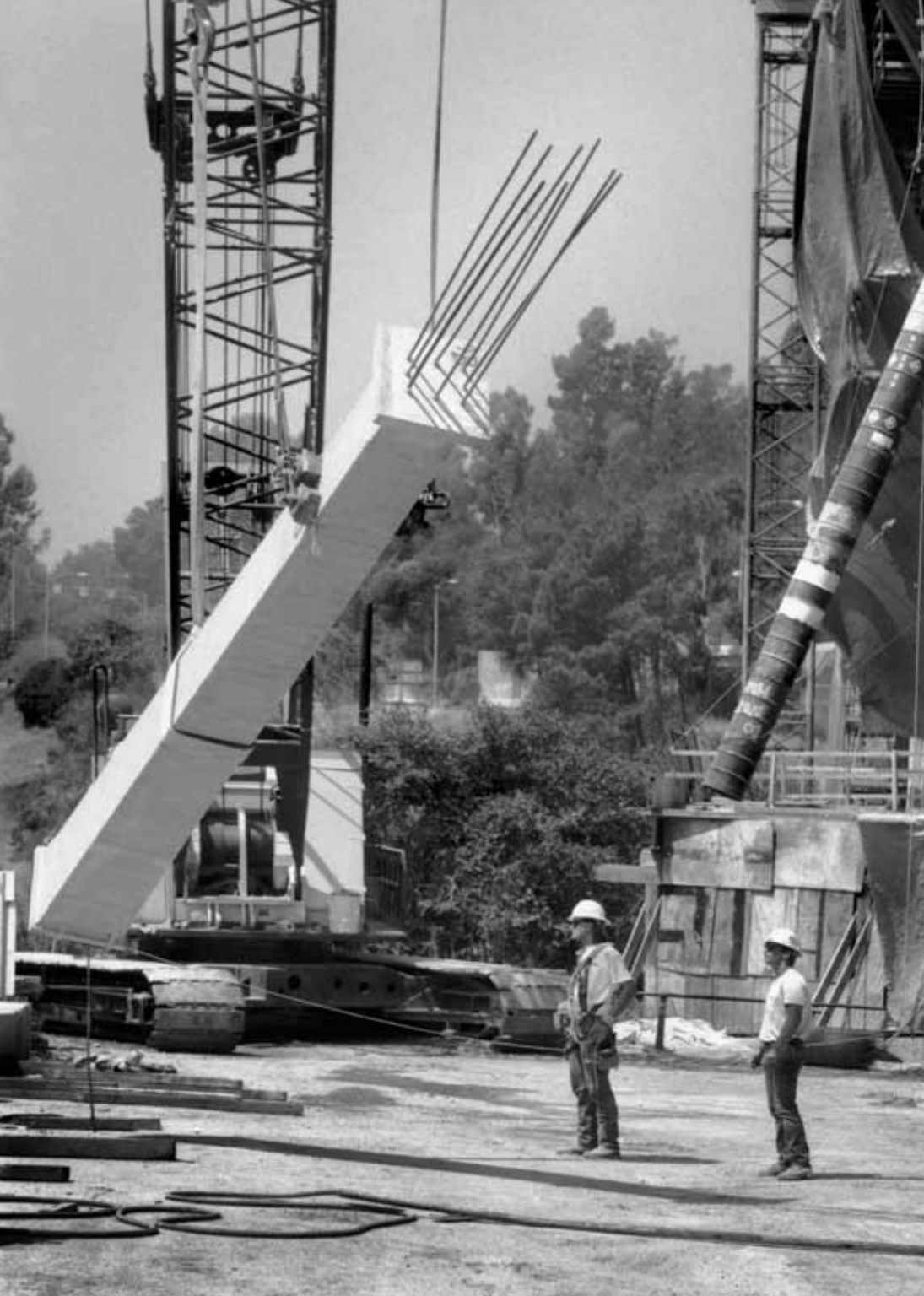
ERECTING NEW PRE-CAST CONCRETE COLUMNS WHICH SUPPORT THE UPPER BRIDGE STRUCTURE.
