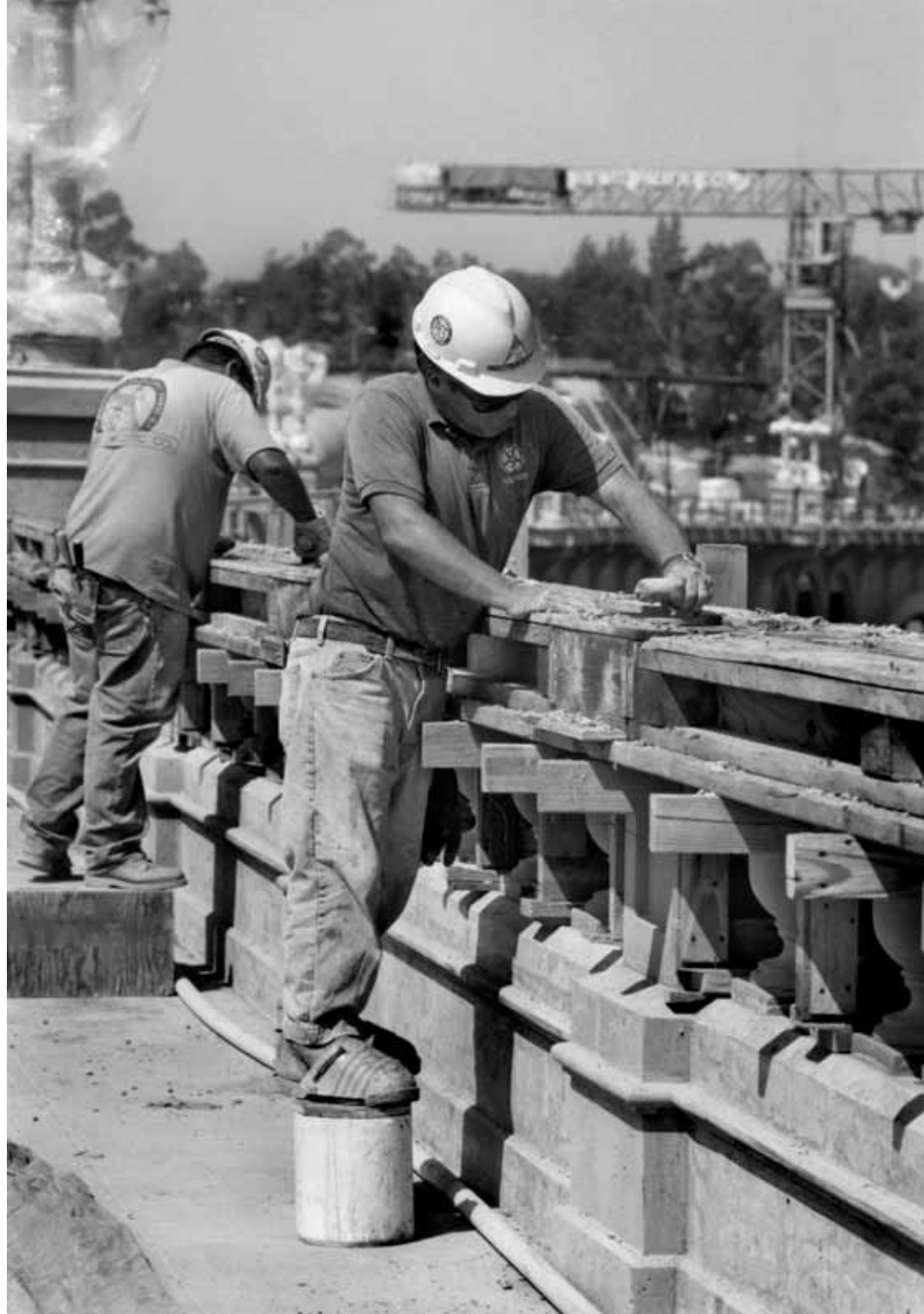
POURING TOP ROW OF BARRIER ROW
