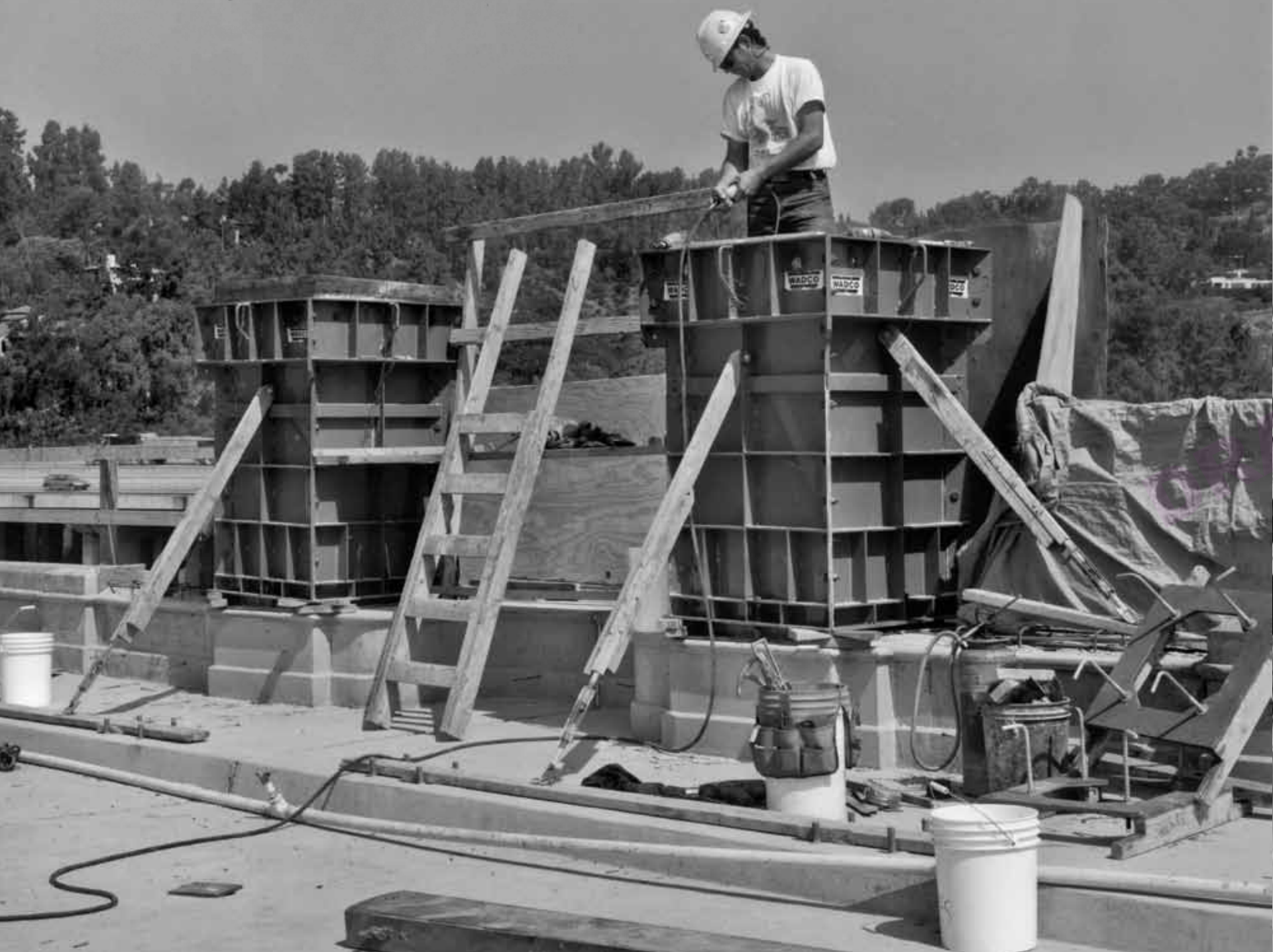
FORMING BASE COLUMNS
