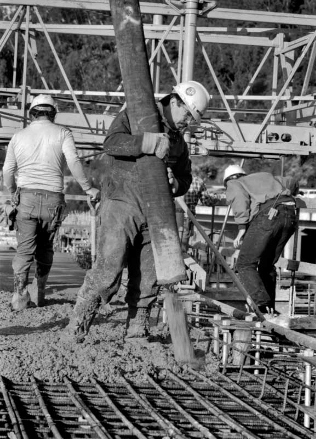
POURING CONCRETE DECK.
