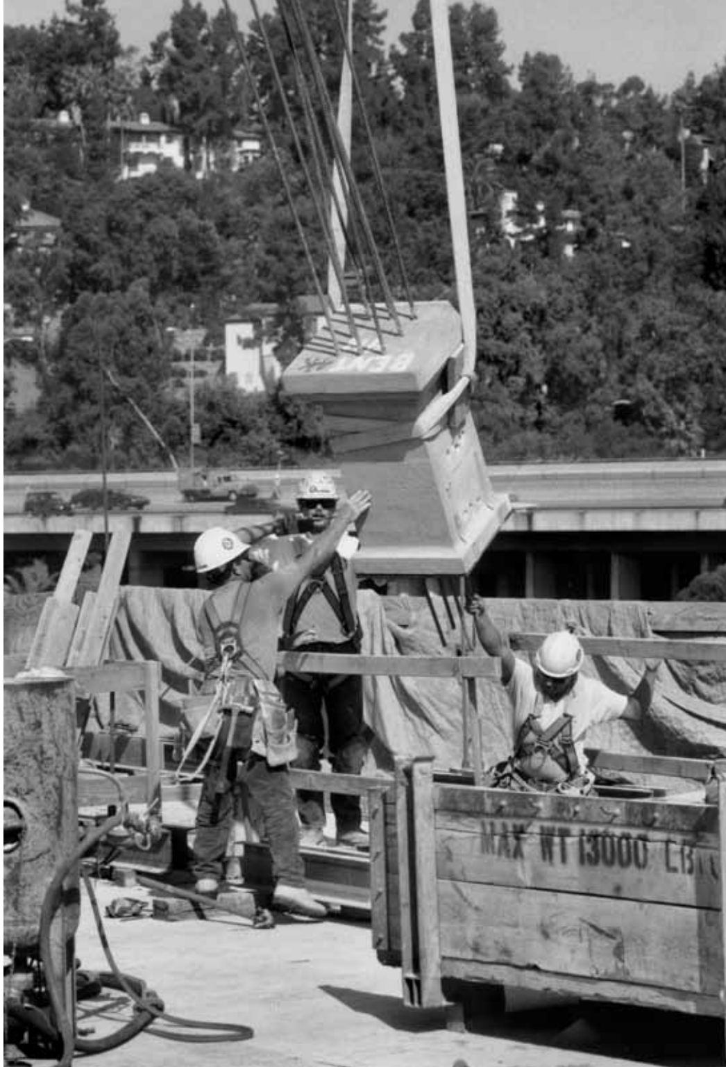
SETTING PRE-CAST CONCRETE PIERS FOR BRIDGE RAIL
