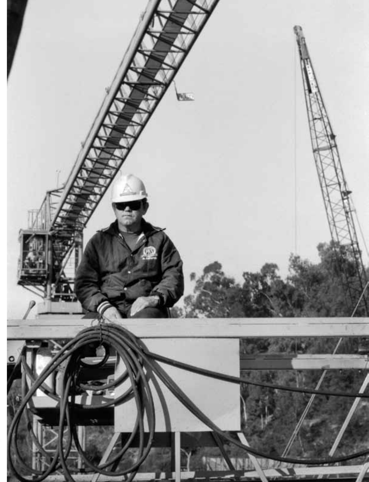
CONCRETE SUPERINTENDENT WATCHING OVER DECK POUR.
